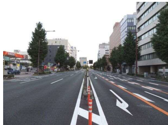
[電線類地中化の施工例]
