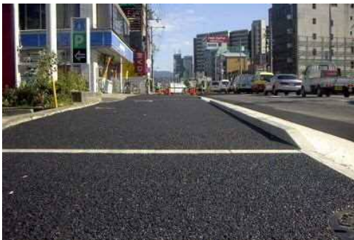
[透水性舗装施工例]
