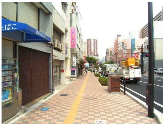
[電線類地中化の施工例]
